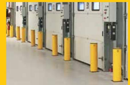
Bollards shielding door frames and shutter runners in a newly built warehousing and distribution center.
