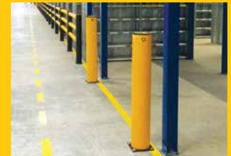
Bollards used to defend entranceway columns in storage facility.
