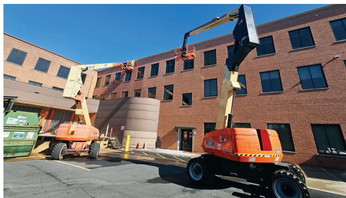
MEWP access avoided full-building scaffolding and disruption.
