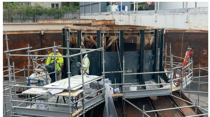
BIG technicians apply SuperWrap II to restore structural integrity.
