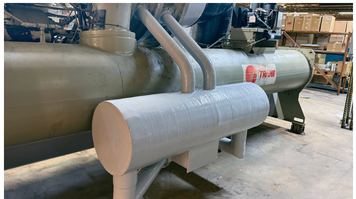
Corroded economizer restored and protected by Superwrap II.
